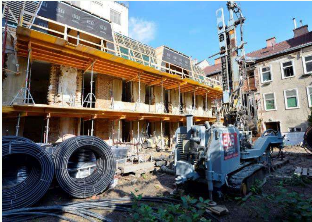
Drilling rig in the inner yard, Source: Gerhard Bayer, ÖGUT
