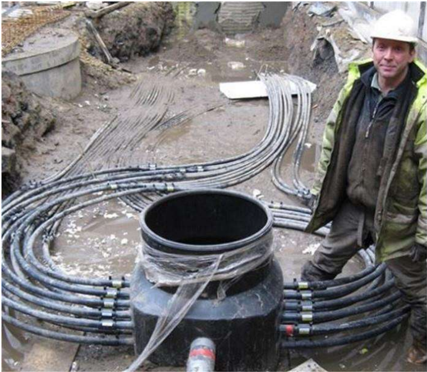
Fusing Connection of pipes with the Manifold Chamber
