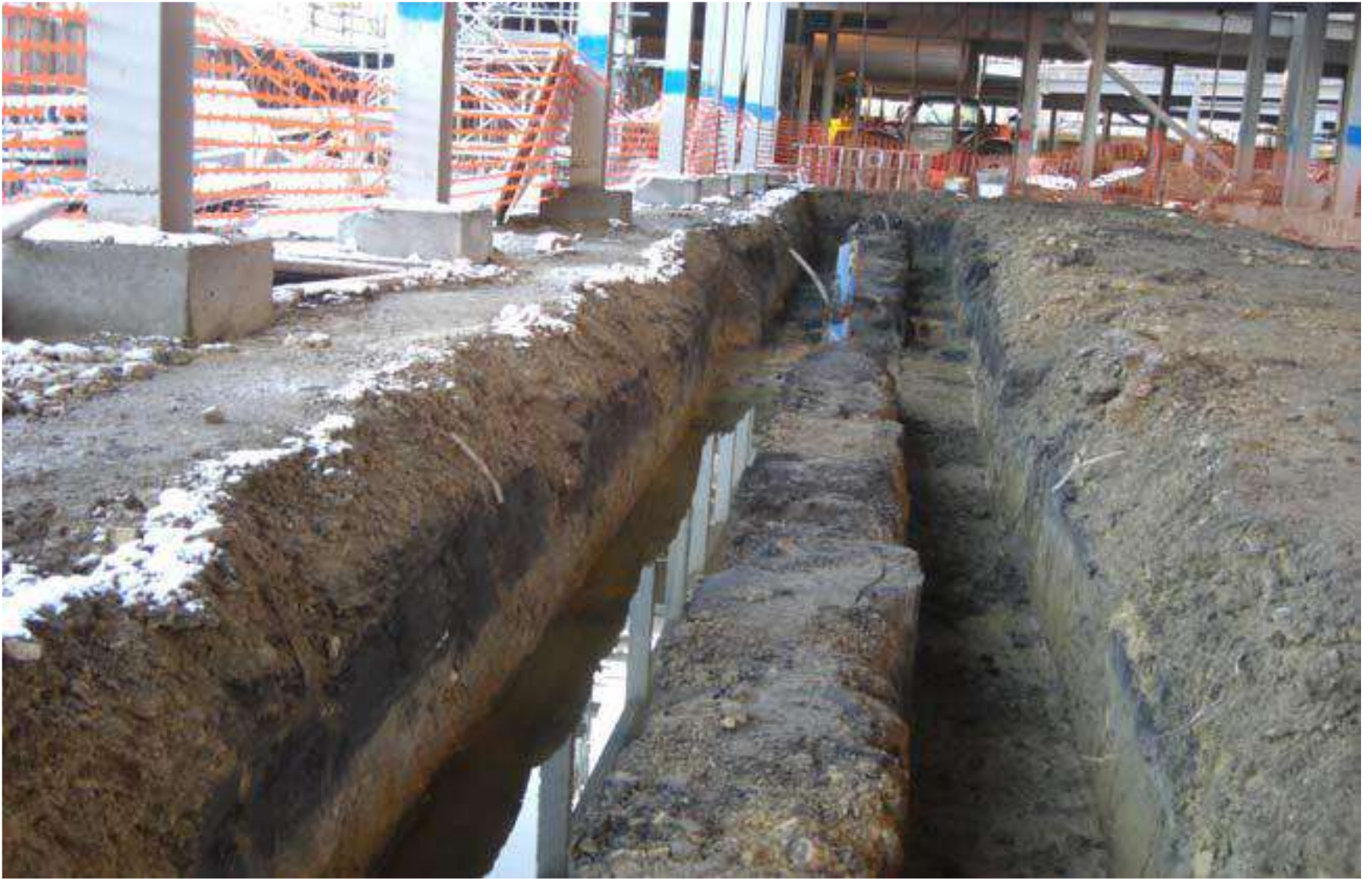
Trenches prepared for connecting heat collector pipes
