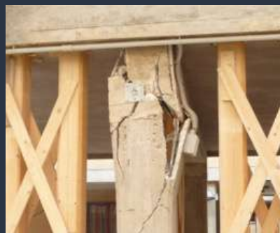
San Salvatore Hospital after the L'Aquila 2009 earthquake Column damage at the main entrance
