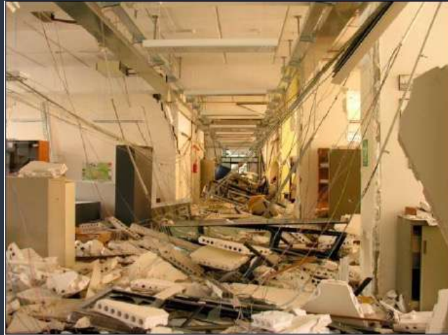
Province building, L' Aquila
