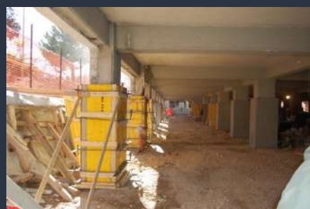
Reinforcement of the substructure's columns
