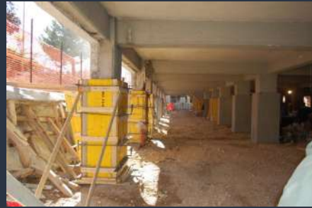
Reinforcement of the substructure's columns
