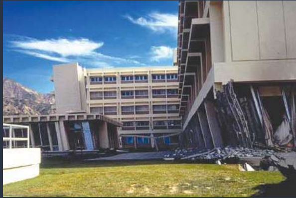
The 1971 San Fernando, California, earthquake (magnitude 6.7) severely damaged the recently built Olive View Hospital
