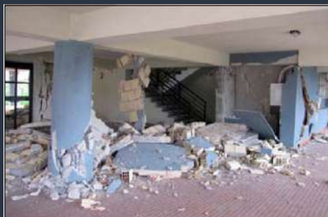
Building in Pettino (AQ)
